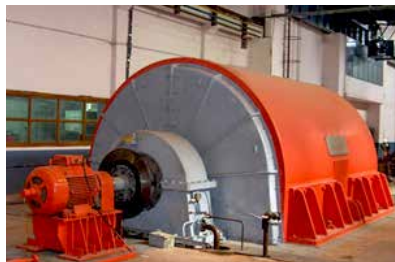
1500MVA Short Circuit Generator
